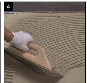
4 Install the tiles Use a flexible adhesive to fix your tiled floor finish directly over the membrane.
