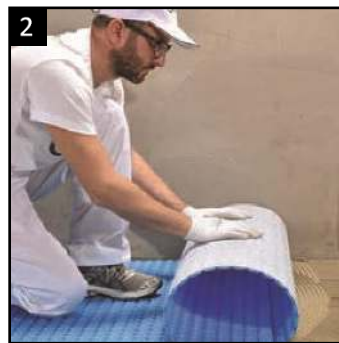
2 Lay the membrane Roll the membrane out over the whole floor and press into the adhesive.
