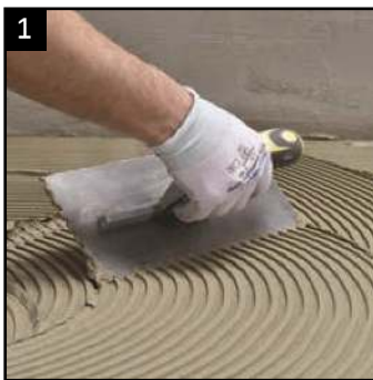
1 Spread tile adhesive Spread a flexible cement based tile adhesive over the floor.
